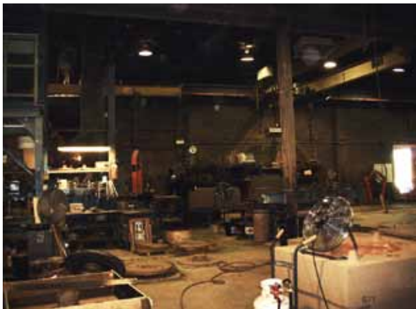
Before lighting upgrade
